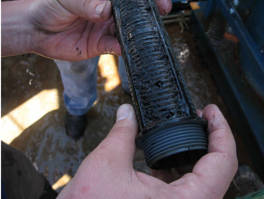
Figure 6-6 Service flow lateral before cleaning for Phase B
